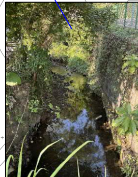
1. Nullah at the entrance of the site
